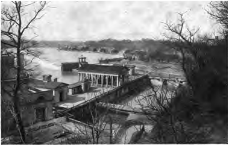
FAIRMOUNT WATER WORKS AND BOAT HOUSE ROW AT THE PRESENT DAY
